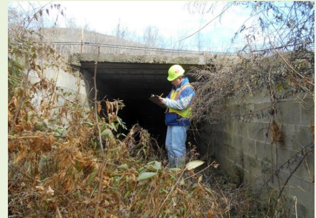
Aboveground structures survey.
